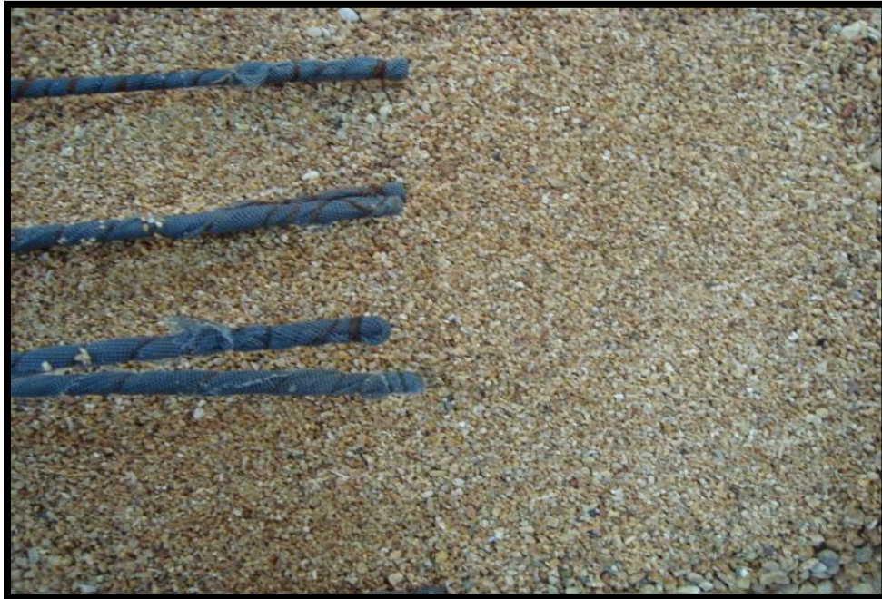
Horizontal drainage blanket with piezometer pipes
